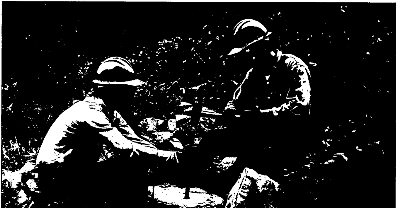
Modified double jacking team at work.
