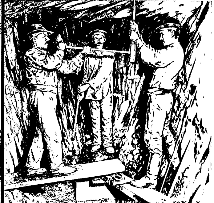
'Up hole' double jacking, early 1800's. (Photos reprinted courtesy of Compressed Air Magazine.)
