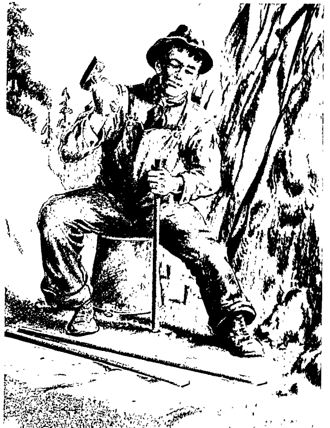
A prospector single jacking, circa 1910. (Photo reprinted courtesy of Compressed Air Magazine.)
