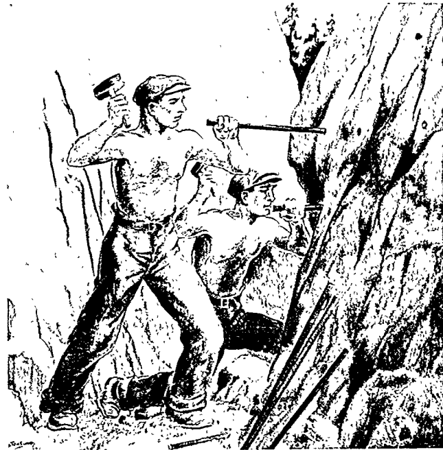
Single jack drilling, circa 1850. (Photo reprinted courtesy of Compressed Air Magazine.)
